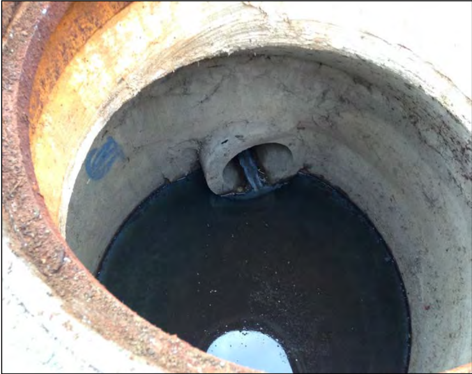
Figure 2: Beech Street Manhole (west of Harvey Street intersection) Sewage Fungus
